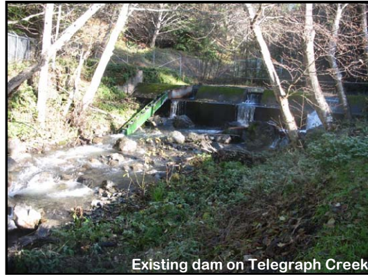
Existing dam on Telegraph Creek
